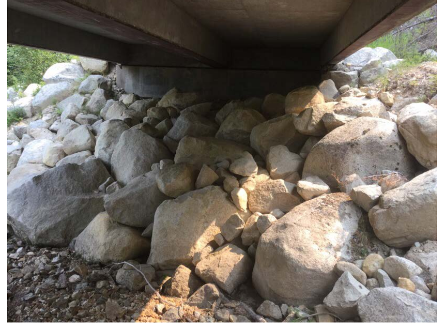
Right Bank Abutment when facing downstream
