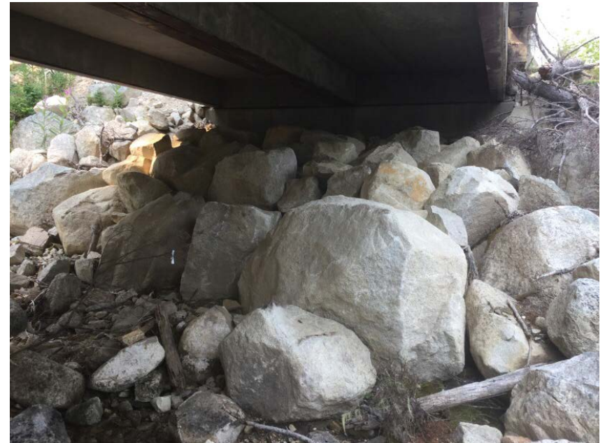
Left Bank Abutment when facing downstream
