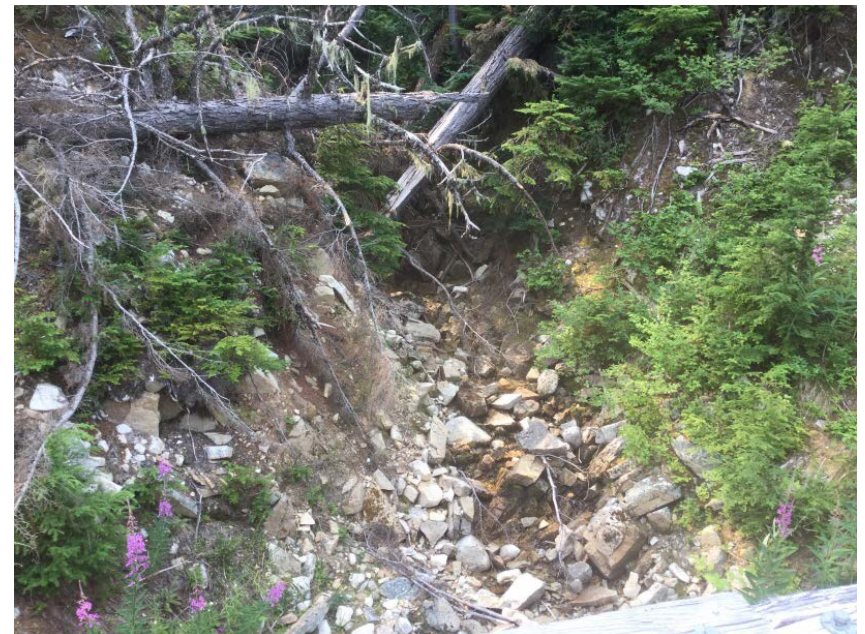
Looking upstream from deck
