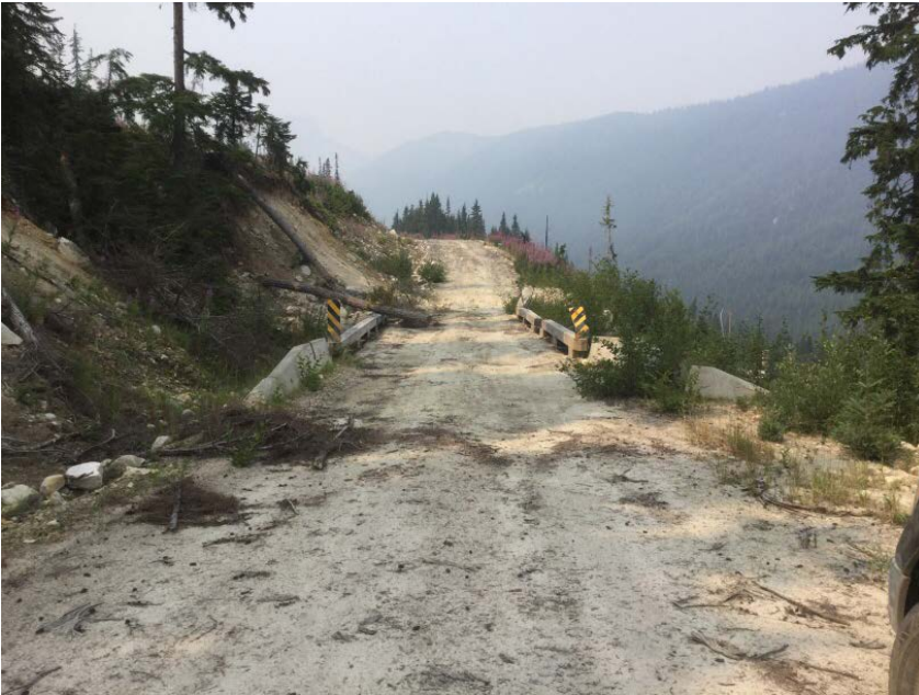
Approach from Right Bank when facing downstream
